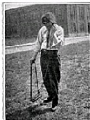
Fig. 2. Proper Method of Handling Exploring Coil When Tracing Path of Pipe.
